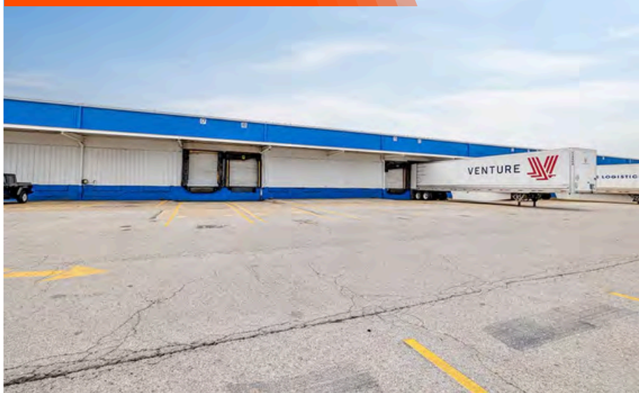
DOCK DOORS WITH LEVELERS
