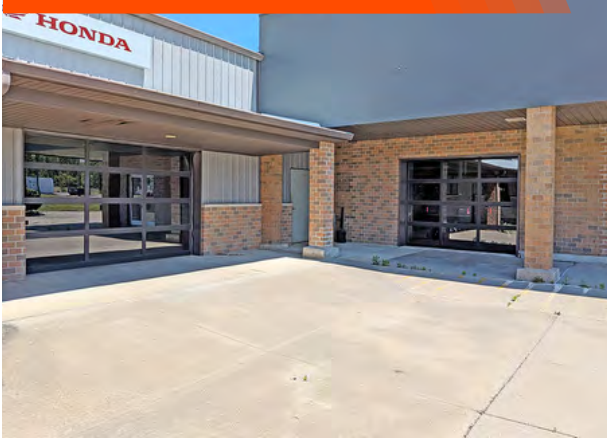
FRONT OVERHEAD DOORS
