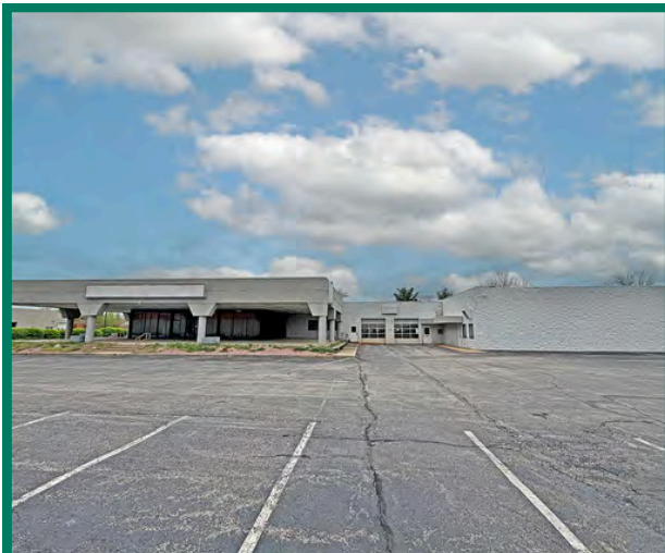
FRONT (2) 10'x10' OVERHEAD DOORS
