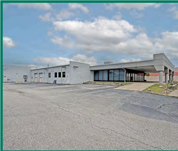
REAR (2) 10'x10' OVERHEAD DOORS
