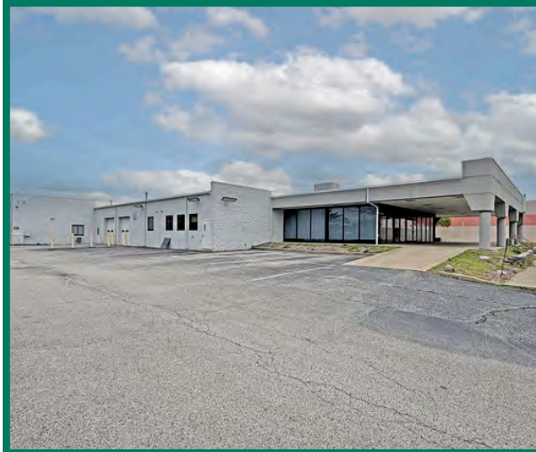
REAR (2) 10'x10' OVERHEAD DOORS
