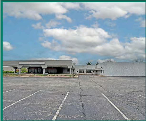
FRONT (2) 10'x10' OVERHEAD DOORS
