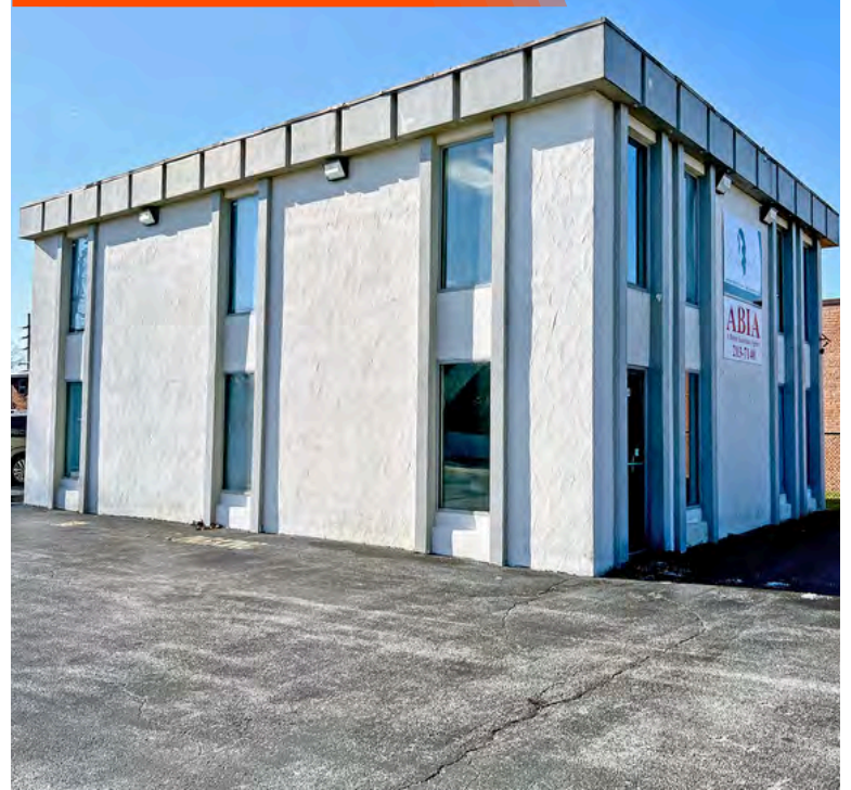
SIDE VIEW EXTERIOR
