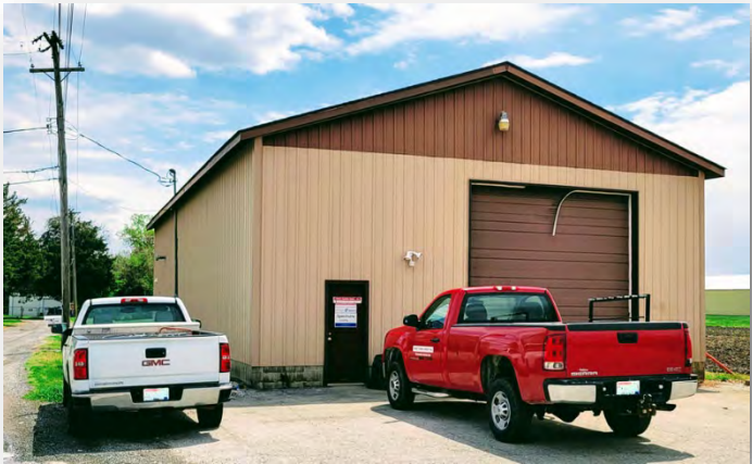
2,800 SF Fully Insulated Shop with 14'x16' Drive-Thru Door.
